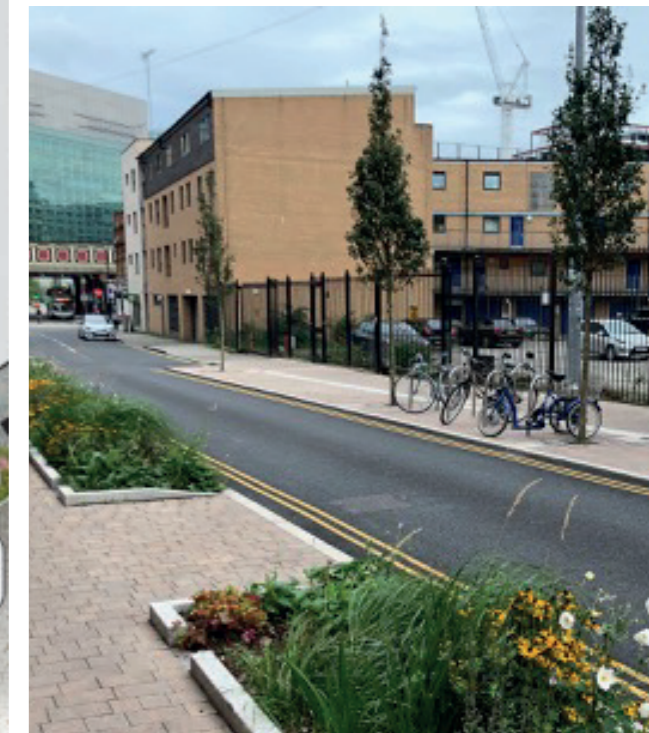
Creating comfortable pedestrian routes and rain gardens / soft planting features making better use of space available
