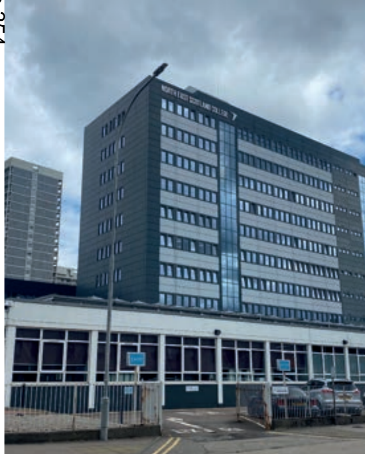
The Masterplan seeks to better integrate NESCOL into the George Street area.
