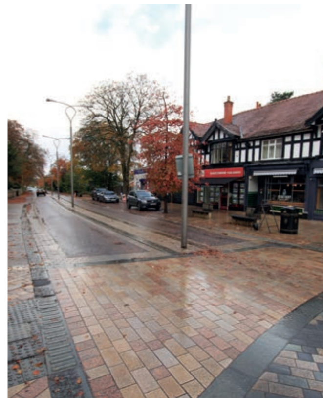
A change in texture and colour can visually narrow the carriageway and slow down traffic
