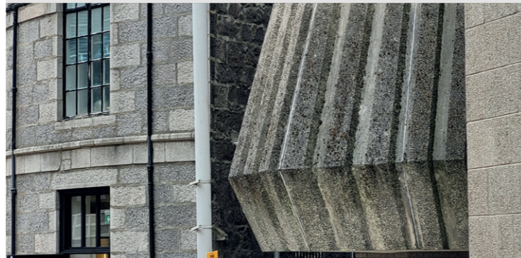
Distinct local character - variety of architecture and materials creating a character to George Street
