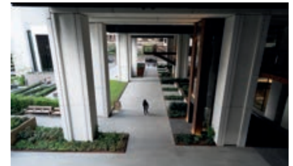
The existing footings and columns of Norco House could be revealed, creating a flowing connection between building and external space
