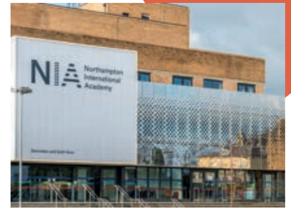
Examples of how an existing building elevation can be screened and enhanced with bold and contemporary materials
